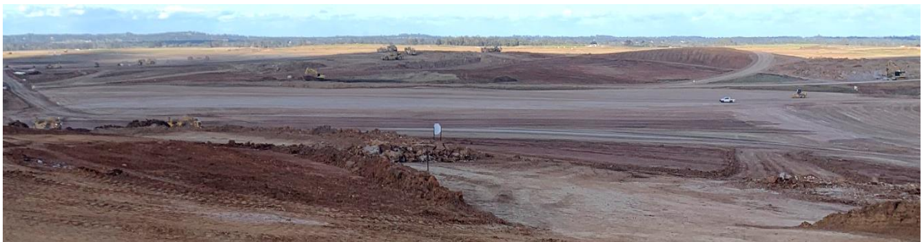
Scrapers working to move 25 million cubic metres of earth at the new airport
