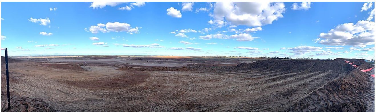
Future 3.7km runway at Western Sydney International (Nancy-Bird Walton) Airport
