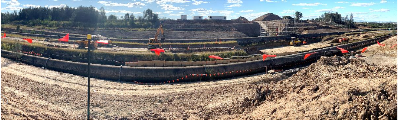
Bridge construction over Water NSW pipelines at Oakdale
