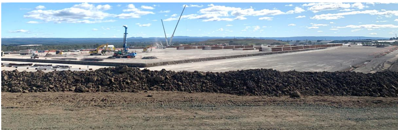
Construction at Oakdale West
